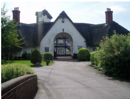
Node Court office in Hertfordshire
